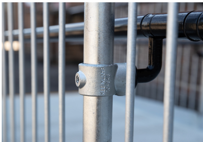
Kee Klamp fittings – Kee Access ramps use tried and tested Kee Klamp fittings for construction
