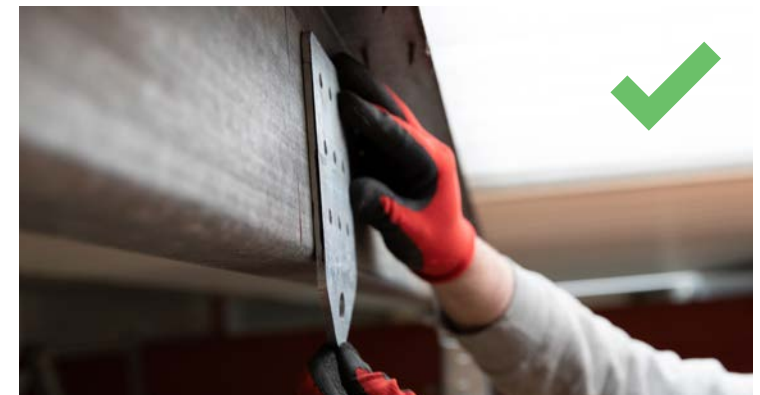
Fig. 2: Correct - bracket bends away from you
