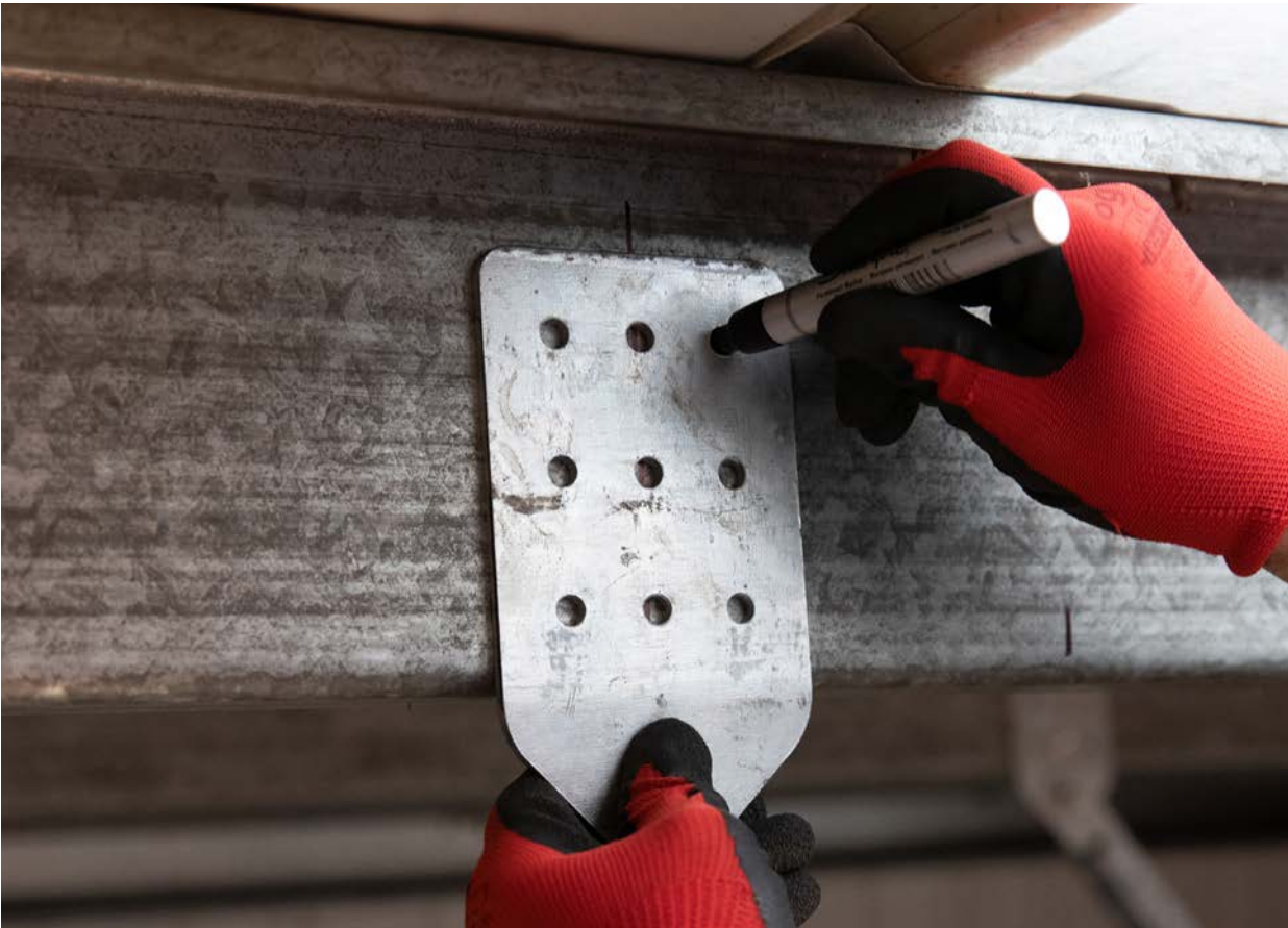
Fig. 1: Incorrect - bracket bends towards you
